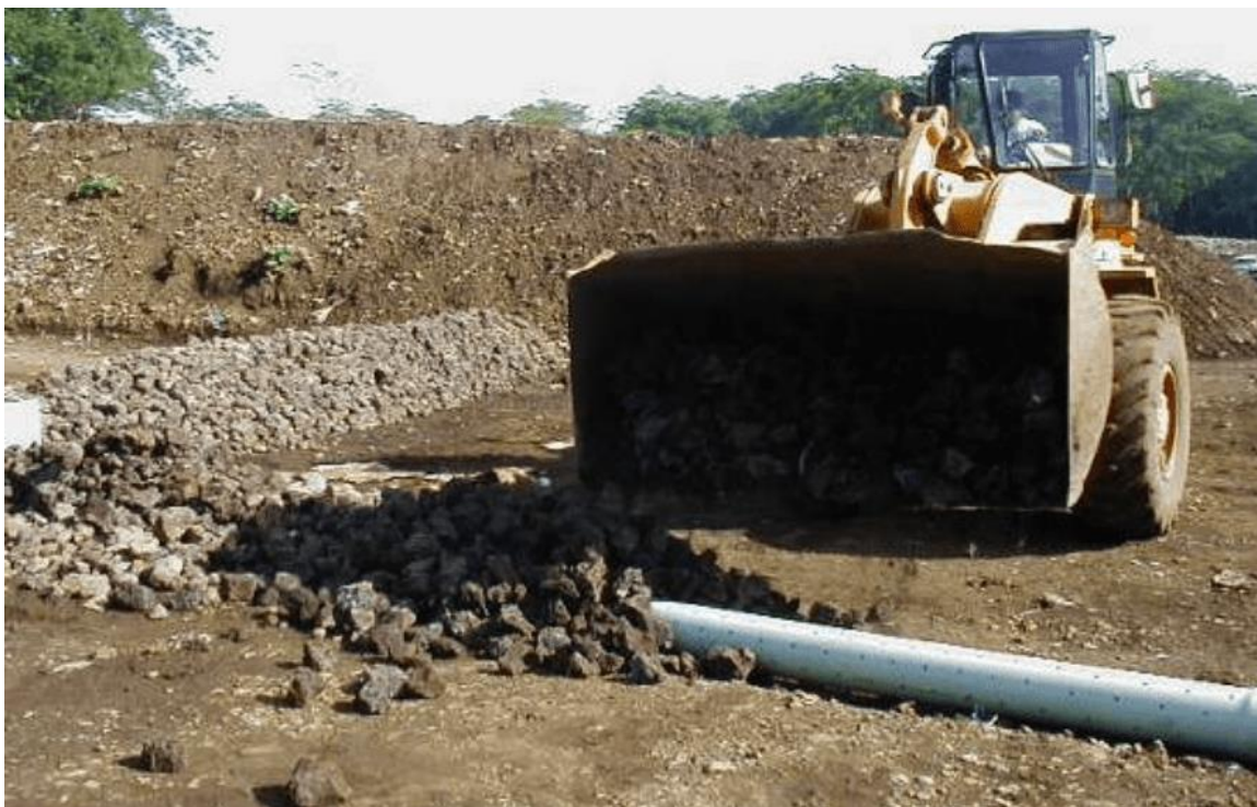
Figure 21 - Installing the leachate line at the base of the site (SPREP, 2010).
