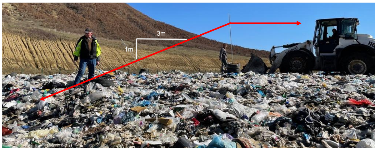
Figure 18 - Example of installing the visual markers on the landfill
